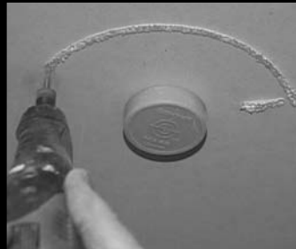
Cut Out Drywall
